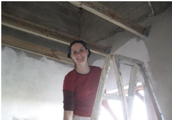
We helped the KwaZulu-Natal mission paint their new buildings and dig out a new septic area.
